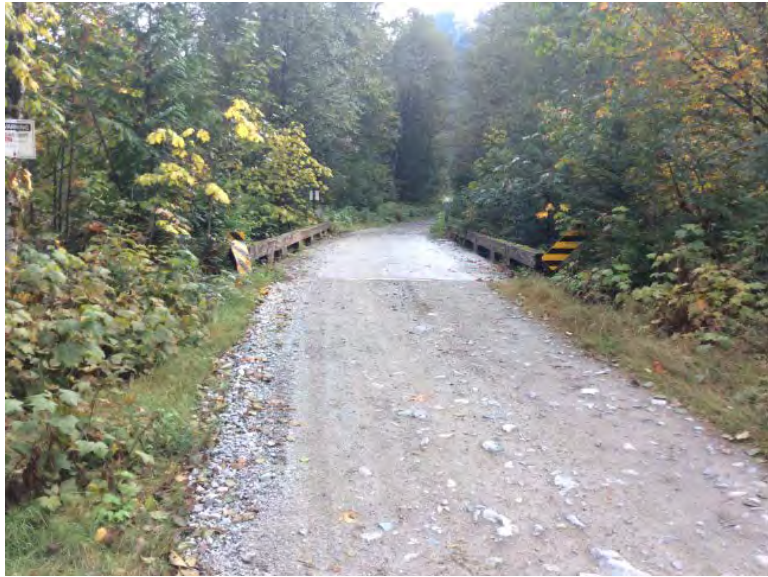
Approach from Left Bank when facing downstream
