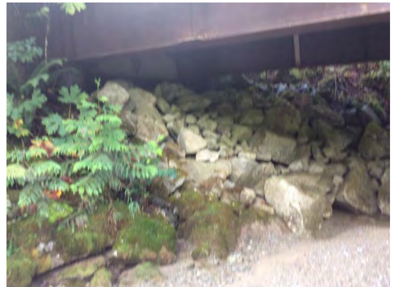
Right Bank Abutment when facing downstream
