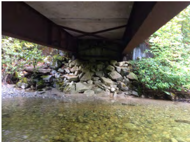
Left Bank Abutment when facing downstream
